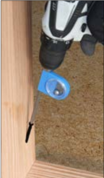
Typical WSTS45-EXT stud to bottom plate installation
