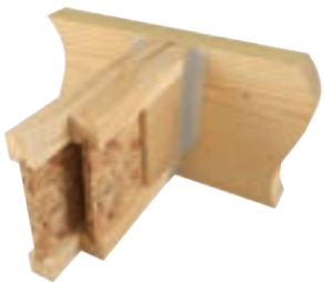
Typical THF double I-Joist installation
