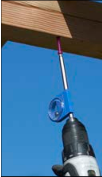
Typical WSTS6-EXT truss to top plate installation
